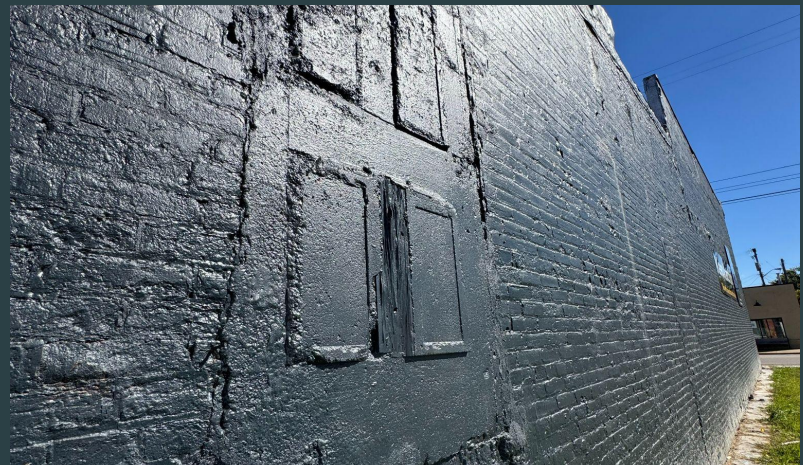
Existing brick + previous repairs
